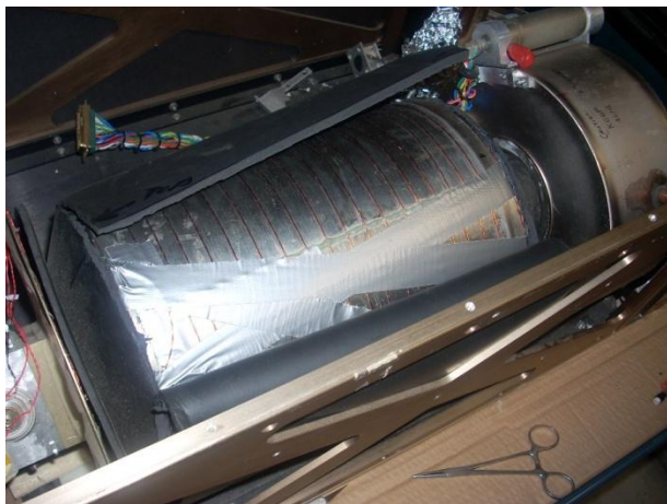
Insulation removal to ID outer oven connects
