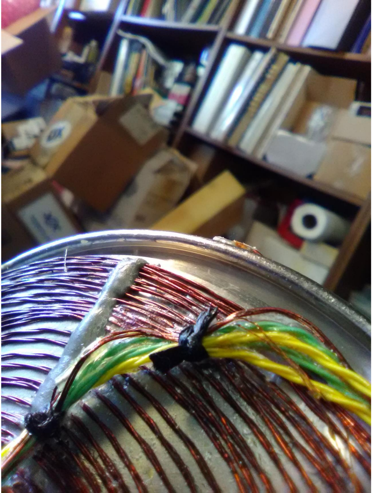
VACUUM ENVELOPE WELD
